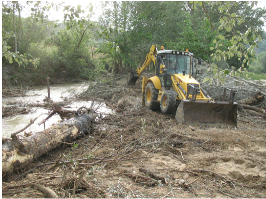
Figure 7. Rebuilding the levee and diverting the river back to its original channel at the divergence point in April 2010.
