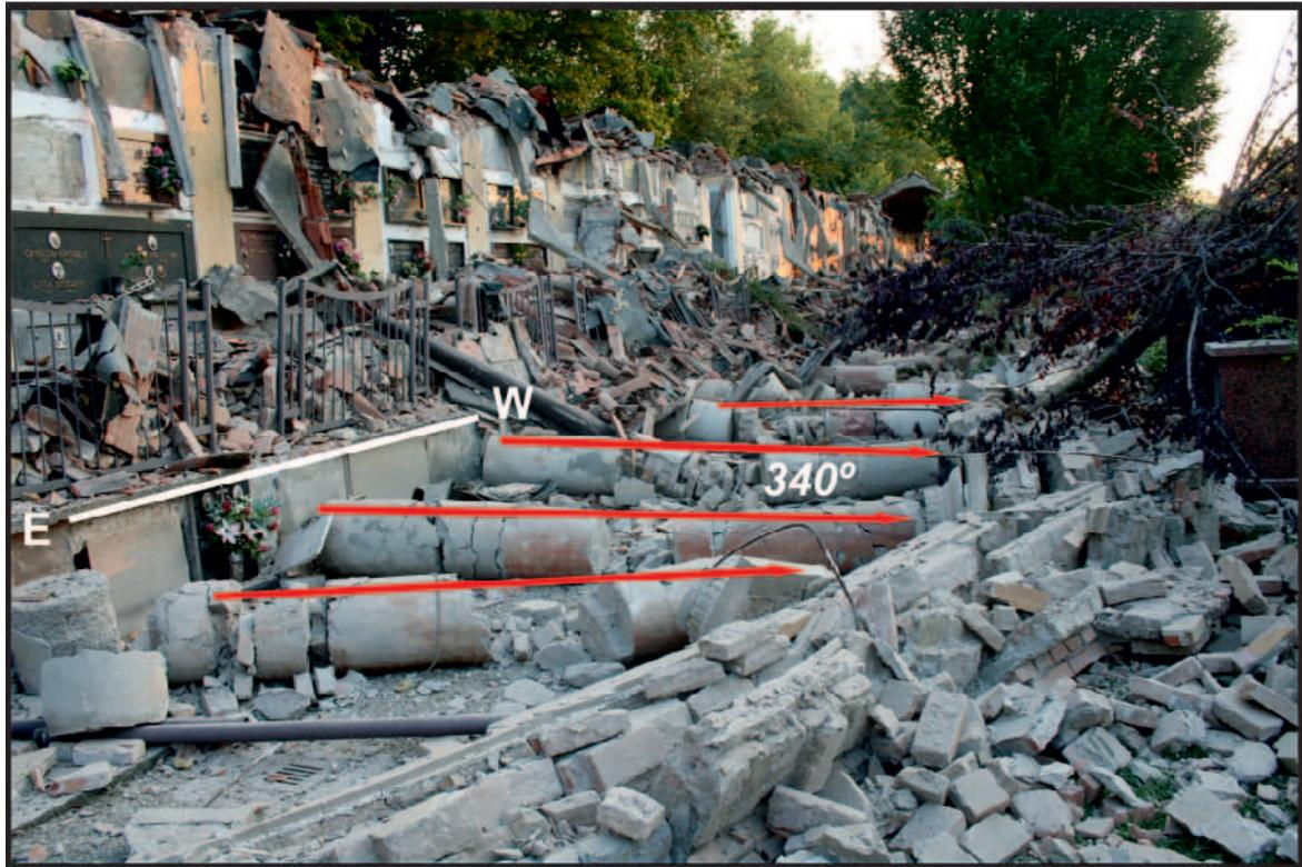
Figure 8. Series of columns collapsed in the cemetery of Mirandola. The azimuth coincides with the displacement vector of the base of the obelisk (see fig.5).
