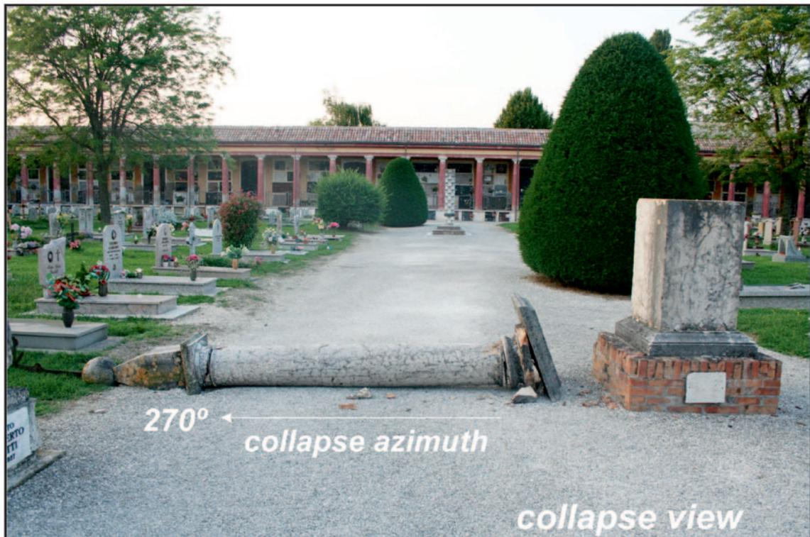
Figure 6. Structure collapsed in the cemetery of Mirandola city (Mai 29 earthquake, Emilia Romagna, Italy). Scheme (a) and photograph (b) of the collapsed structure. The obelisk collapses towards the N270°, while the base undergoes rotation and displacement (N340°).
